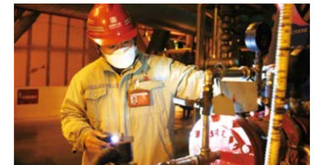
Enhanced regular checks of equipment
