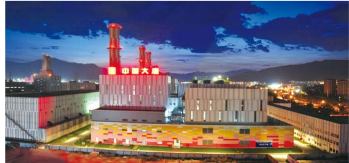
Beijing Gaojing Thermal Power Plant has two gas-steam combined cycling units with installed capacity of 1,380 MW currently. It is the largest gas plant under China Datang Corporation in service and in Beijing.
